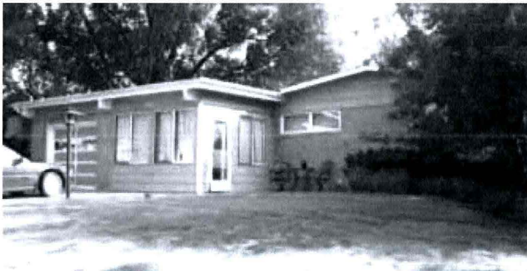
Figure 71. Ranch house in National Register-eligible Eastridge Historic District in Lincoln, Nebraska, constructed c.1953; one of several homes with an altered garage that is considered contributing (Mead & Hunt photograph)
